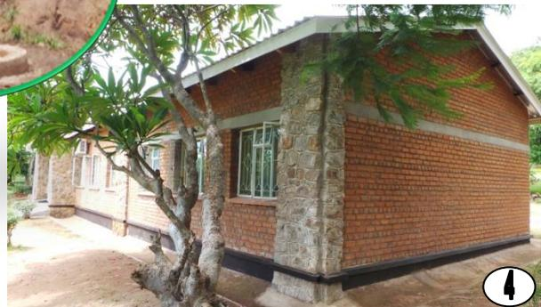
1: The Front view of the kitchen and dining hall. It shows the newly constructed extension conference room attached to the main hall. It also shows two air conditioners newly installed and the roof painted with roof guard to protect the iron sheets from rust.
